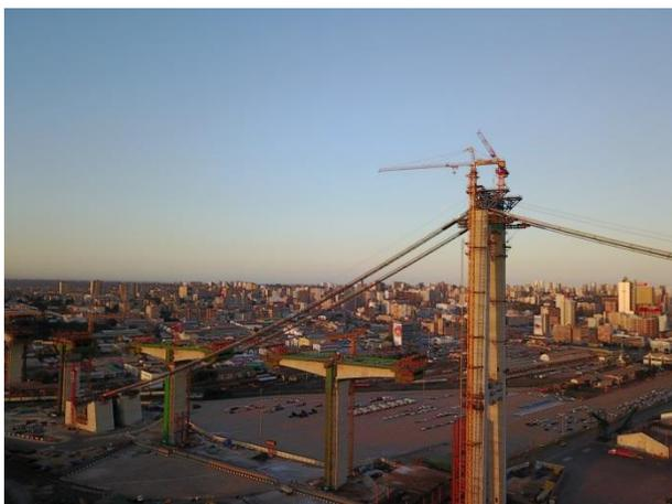
Figure 4: North pylon and free cantilever bridge
