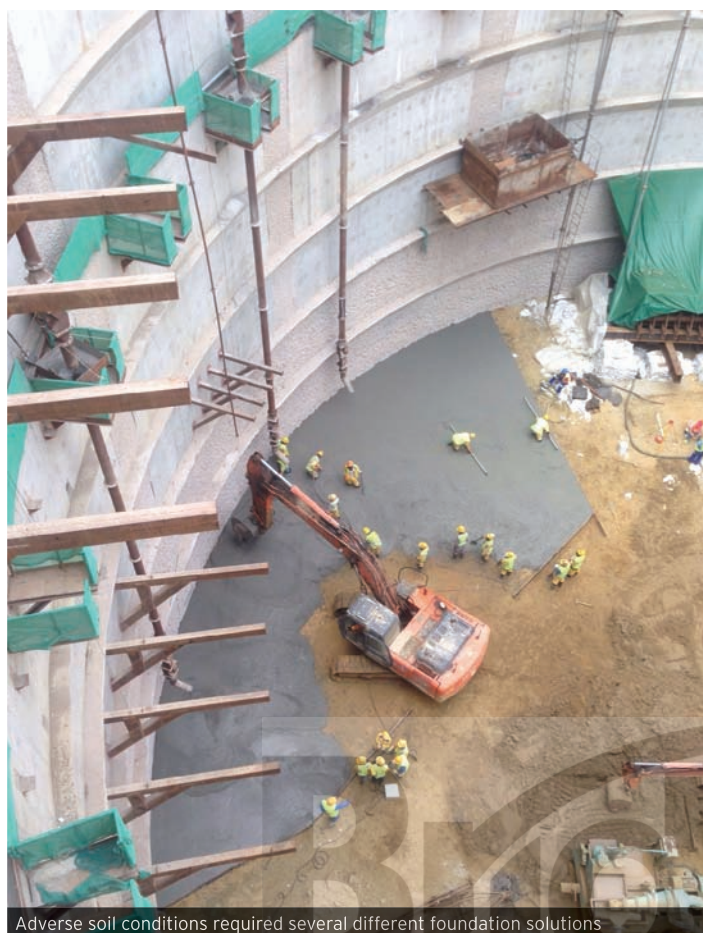
Adverse soil conditions required several different foundation solutions
