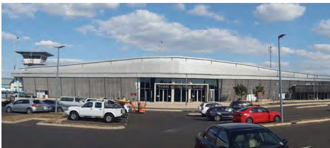
Kasane International Airport Terminal Building, Botswana Project Management and Construction Winner - SAICE Johannesburg Awards 2017
