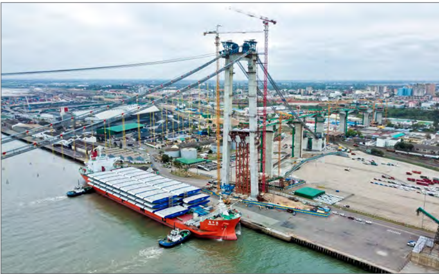
The girders will be lifted off the ship, rotated into place and attached by hangers to two 0.509 m diameter galvanised 91-strand cables; each segment will then be connected to the next, and specialist-welded into place
