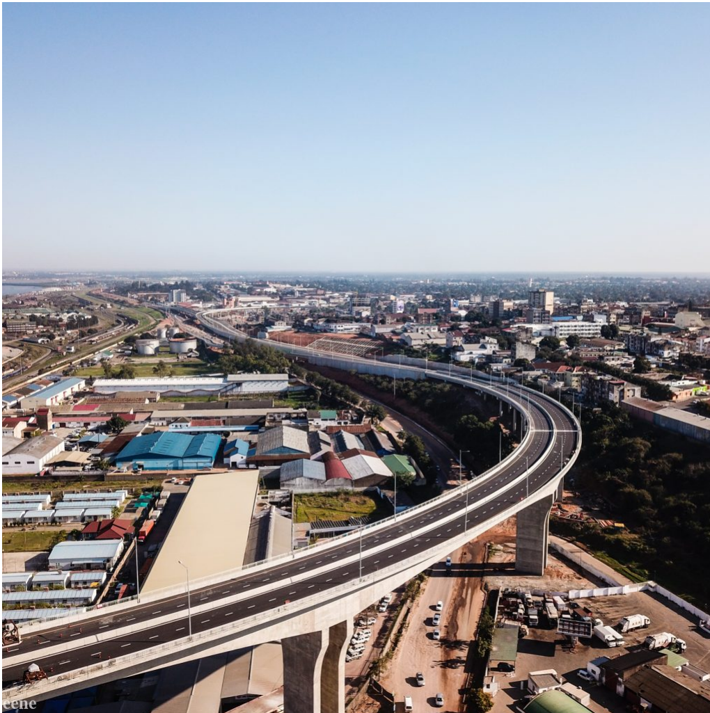
Maputo Bridge North approach
