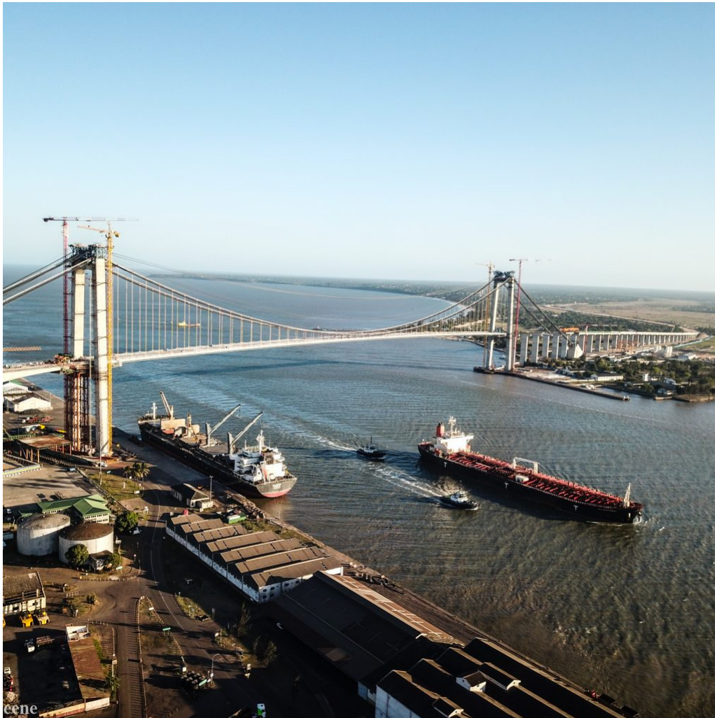
Maputo Bridge Mid span
