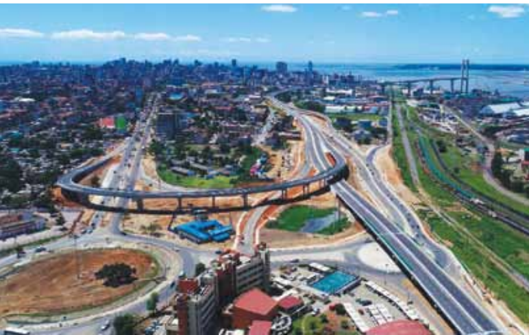
Bridge and ramps of 978 m to North Approach Bridge.
