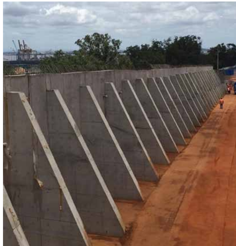
Large retaining wall of the N-Ramp.
