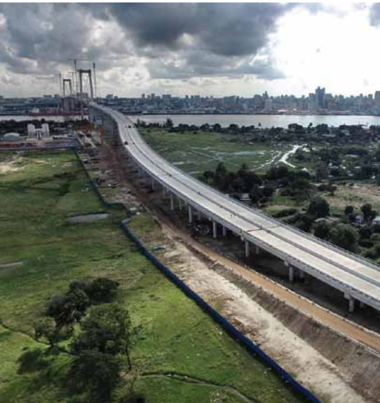
A total of 1234 m of T-beams connect Katembe to Main Bridge.
