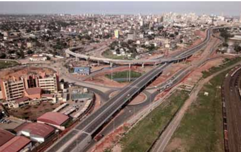
K-Ramp and K-Line going from National Road EN1.
