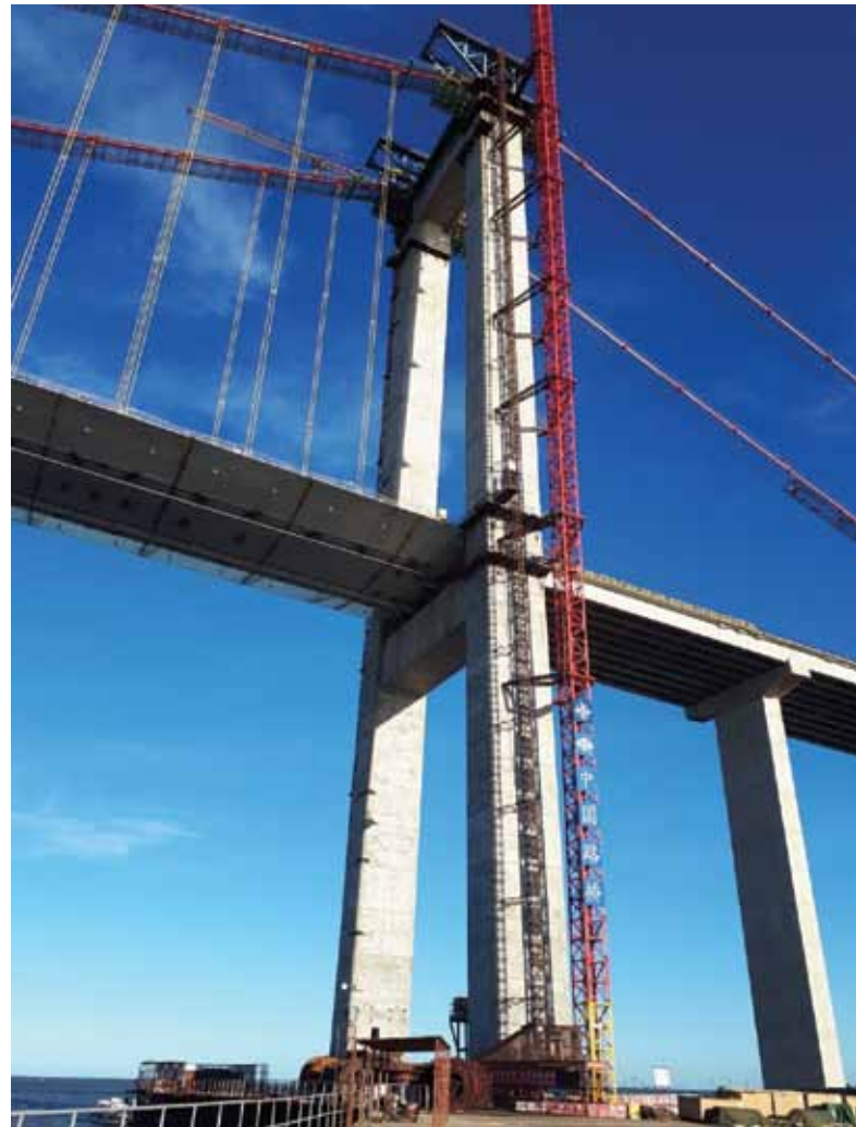
South Pylon - the tallest structure in Maputo (138 m).
