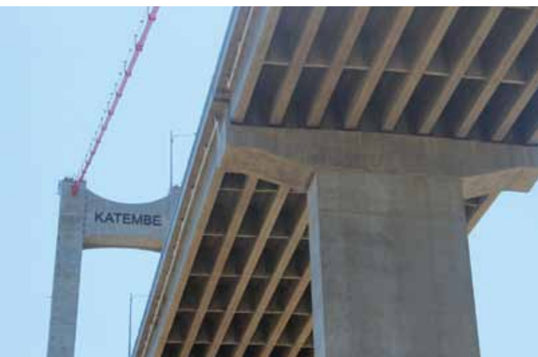
Post-tensioned 45 m-long T-beams connect to Pylon M2.
