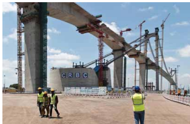
Free cantilever bridge (spans < 119 m) and the northern anchor block.
